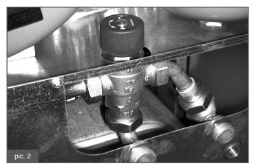
When the boiler is in **"warm boiler ON**" mode ( I led ON), the primary heat exchanger, when CH or DHW are not required, is kept to a constant 50°C temperature.
